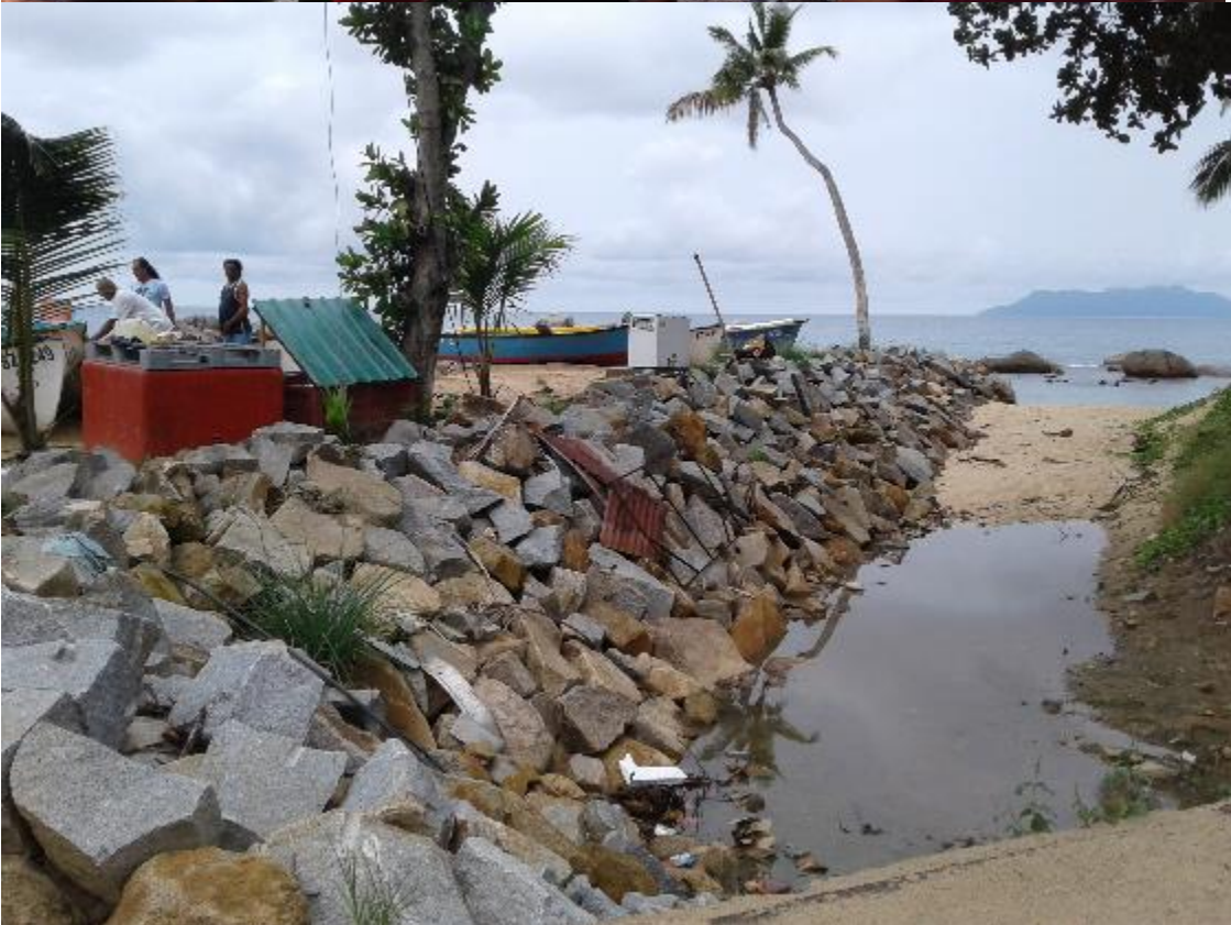
Top: Ex Bel Ombre DA Pharisianne Lucas explaining what happened when the river flooded at Mont Simpson in 2014. Bottom: river outlet rock revetment at Glacis.
