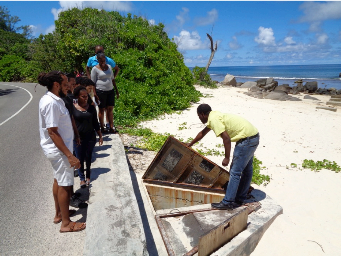
Inspecting a drainage infrastructure opposite the marsh under rehabilitation (Under EBA project)
